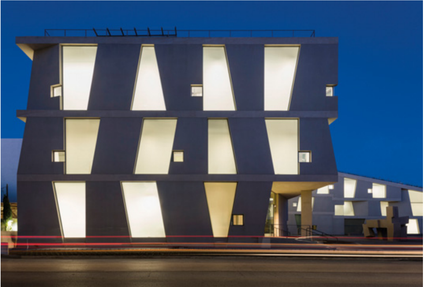
Night view of the Glassell School of Art, west elevation.
